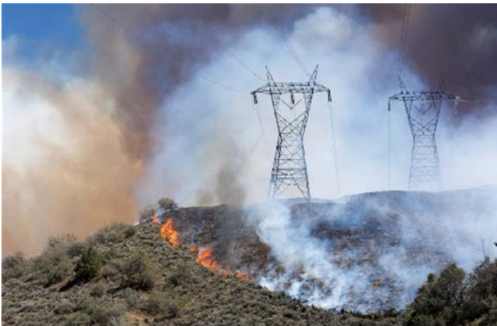
A wildfire burns near utility transmission lines in Southern California.
