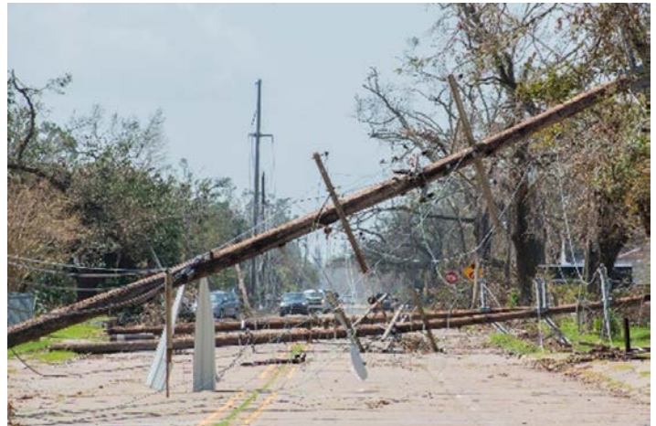
Damage from Hurricane Laura, which struck Louisiana in August 2020.
